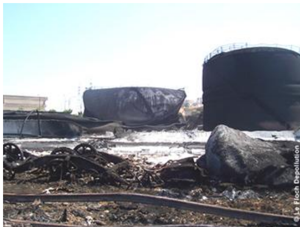
Storage tank of the Jieh power plant after the bombings in July 2006 ©LE FLOCH DEPOLLUTION
