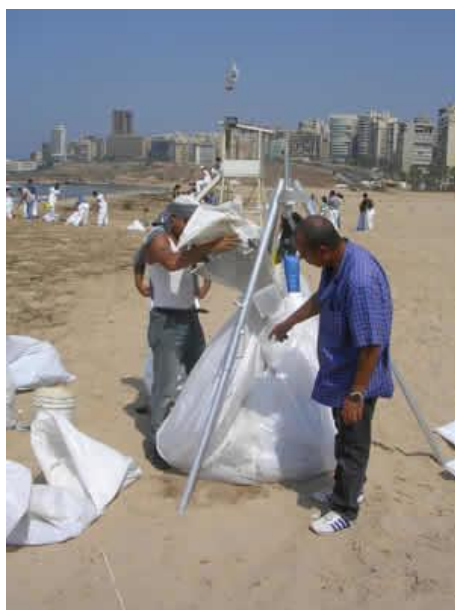
Depollution work site, Ramlet al Baida, September 2006 ©CEDRE
