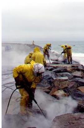
Cleaning riprap with high-pressure cleaners ©CEDRE
