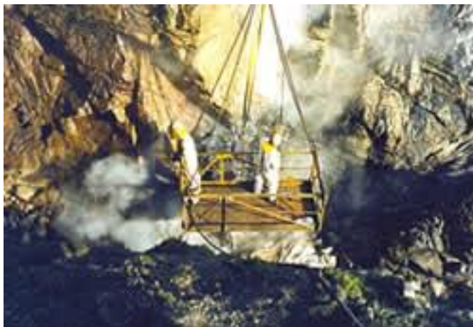
High-pressure cleaning of cliffs at the FOSELEV/SIS worksite (Loire-Atlantique) ©CEDRE
