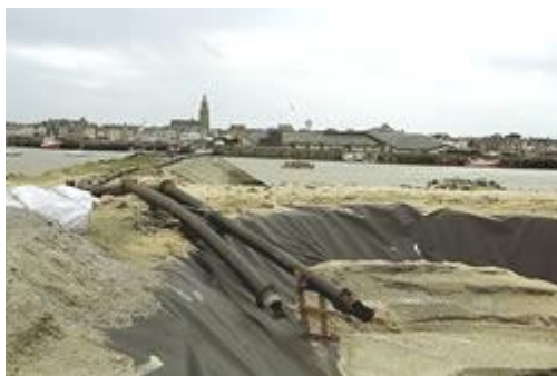
Separation trenches for the collected waste ©CEDRE
