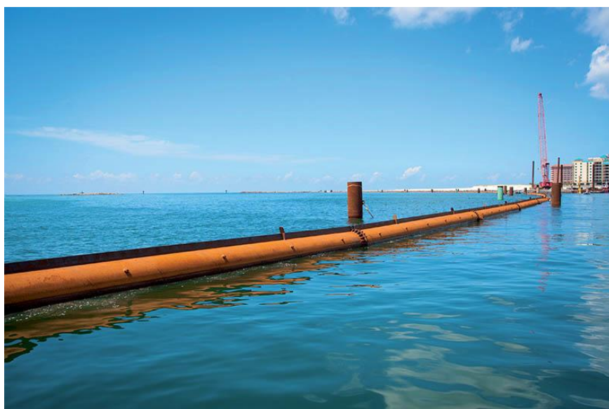
Rigid Tube Boom: floating booms fixed to spikes ©USCG PHOTO
