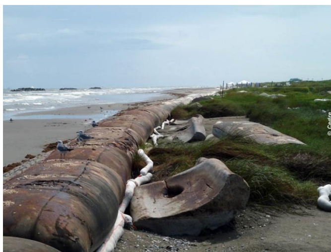
Anti-erosion system and sorbent booms ©CEDRE
