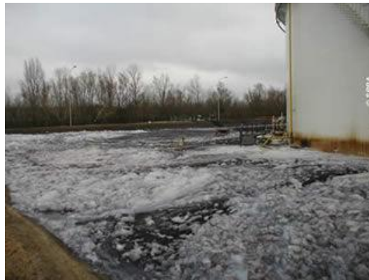
Foaming agent sprayed in the retention tank ©CEDRE
