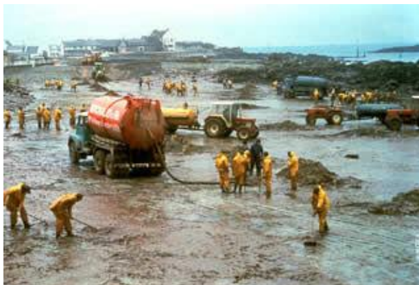
Manure tanks used to store the oil pumped on the shoreline ©NOAA
