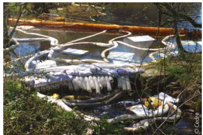
Water level control system and oil containment system at the weir of the first pond
