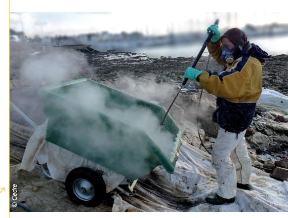
Thermal washing of pebbles in a wheelbarrow protected by geotextile
