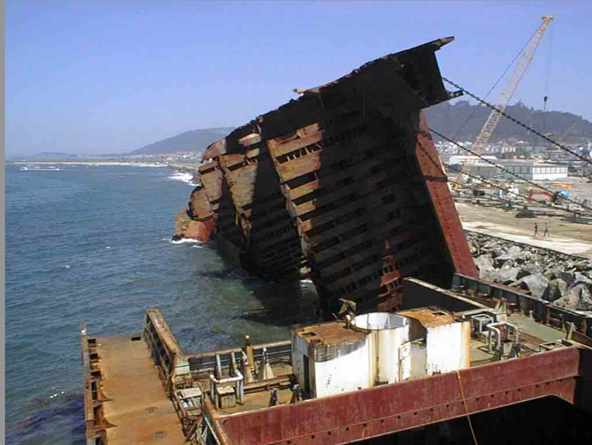
PULLING FORWARD SECTION WITH 9 CHAINS/PULLERS.
