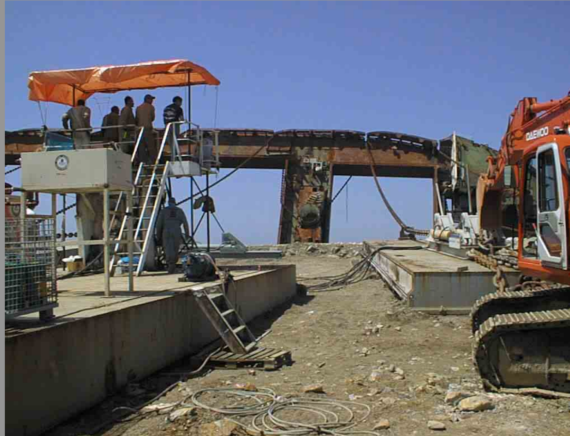
PULLING FORWARD SECTION WITH 9 CHAINS/PULLERS.
