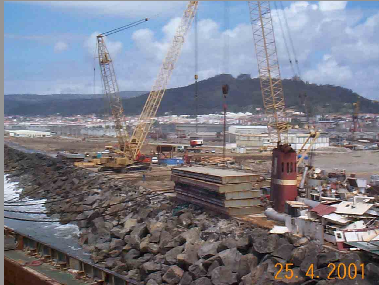
EXTENDED BREAKWATER SITE, SHOWING TWO HEAVY LIFT CRANES IMPORTED FROM UK.
