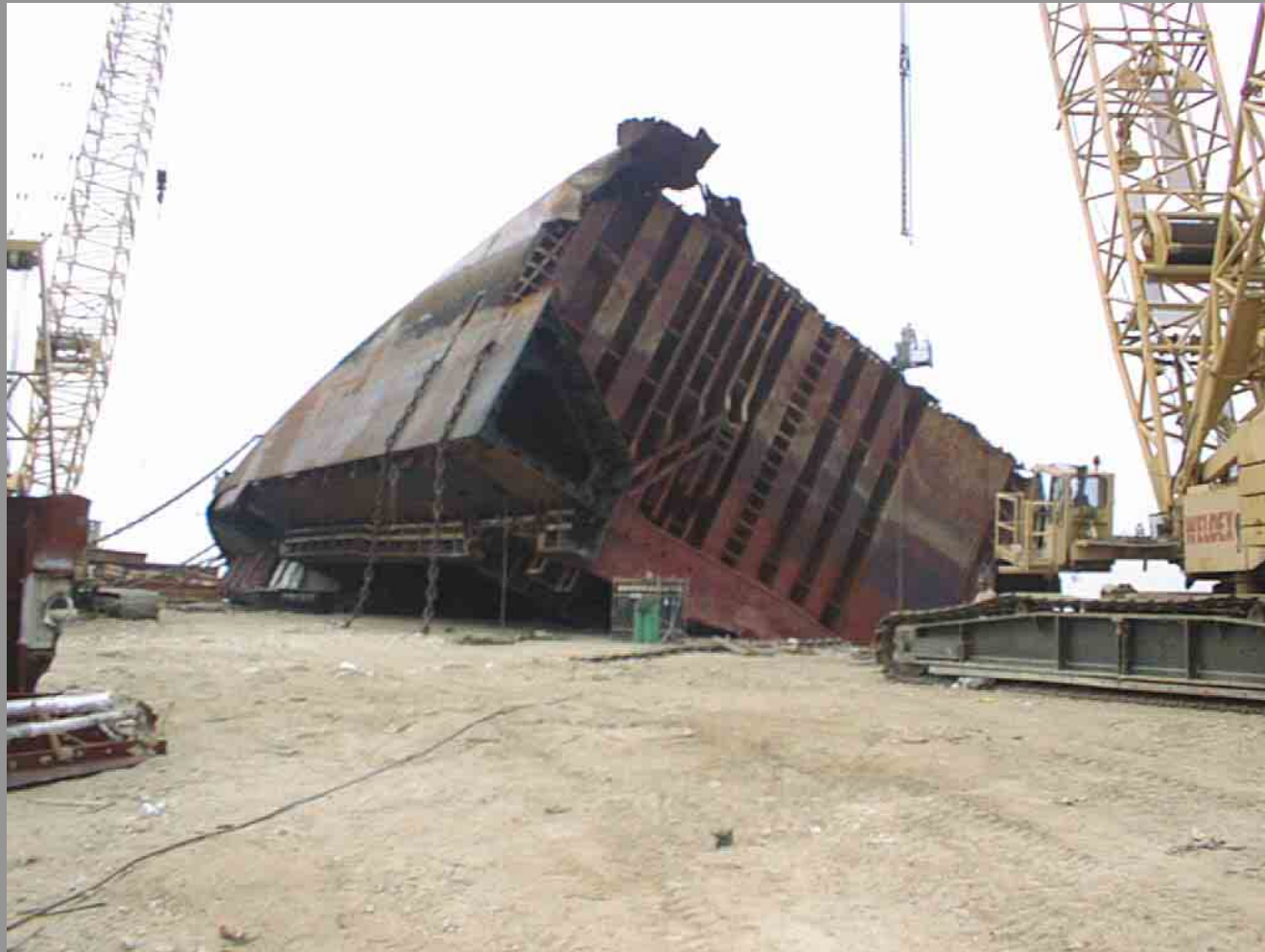
STERN SECTION ROLLED ONTO BREAKWATER
