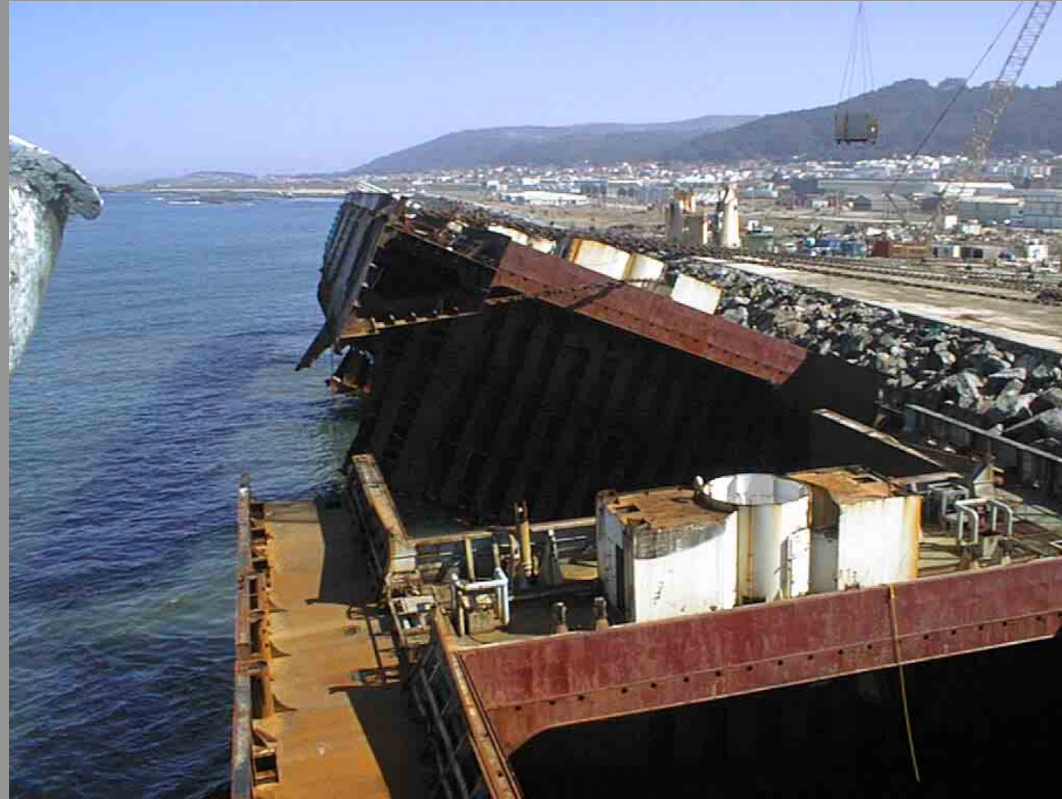
PULLING FORWARD SECTION WITH 9 CHAINS/PULLERS.
