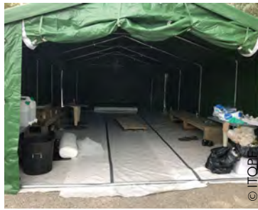
Example of worksite equipment
