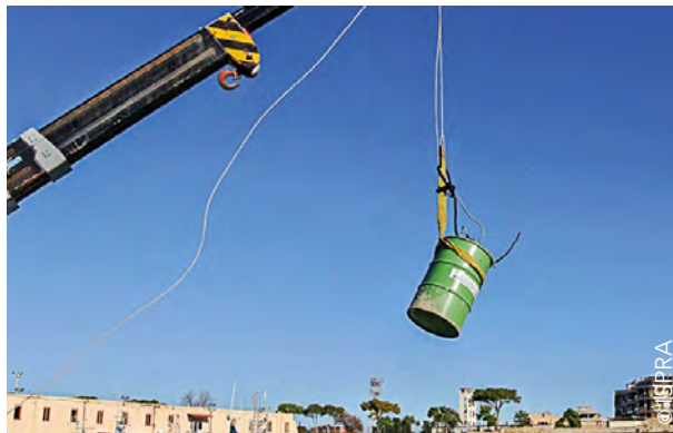
Lifting a drum with a crane
